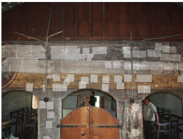
Fig. 12. Nave (separating wall of the nave and narthex)
