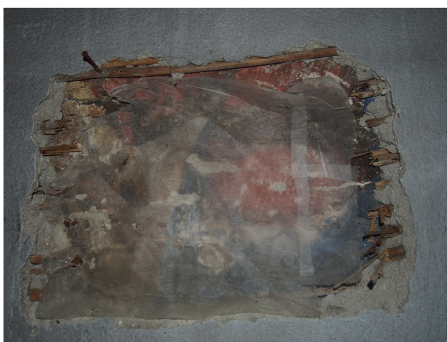
Fig. 11. Narthex (the old painting under mortar again)
